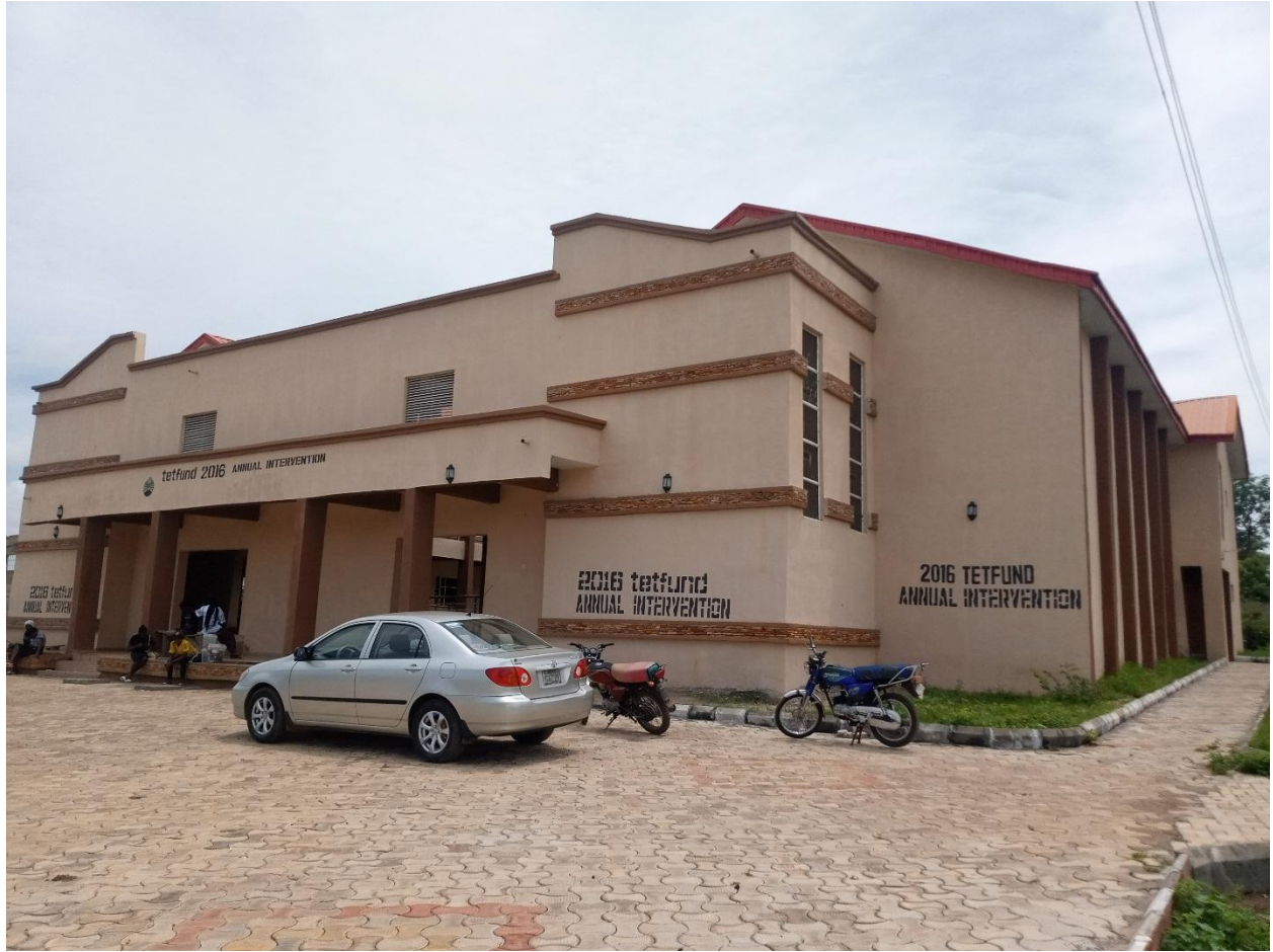
Tetfund 2016 6 Nos of Lecture Rooms with Offices
