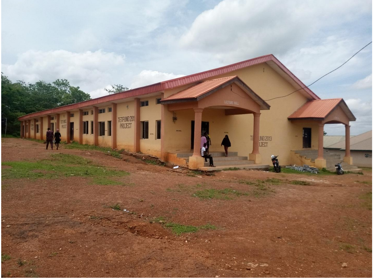
Tetfund 2013 400 Seating Capacity Lecture Hall
