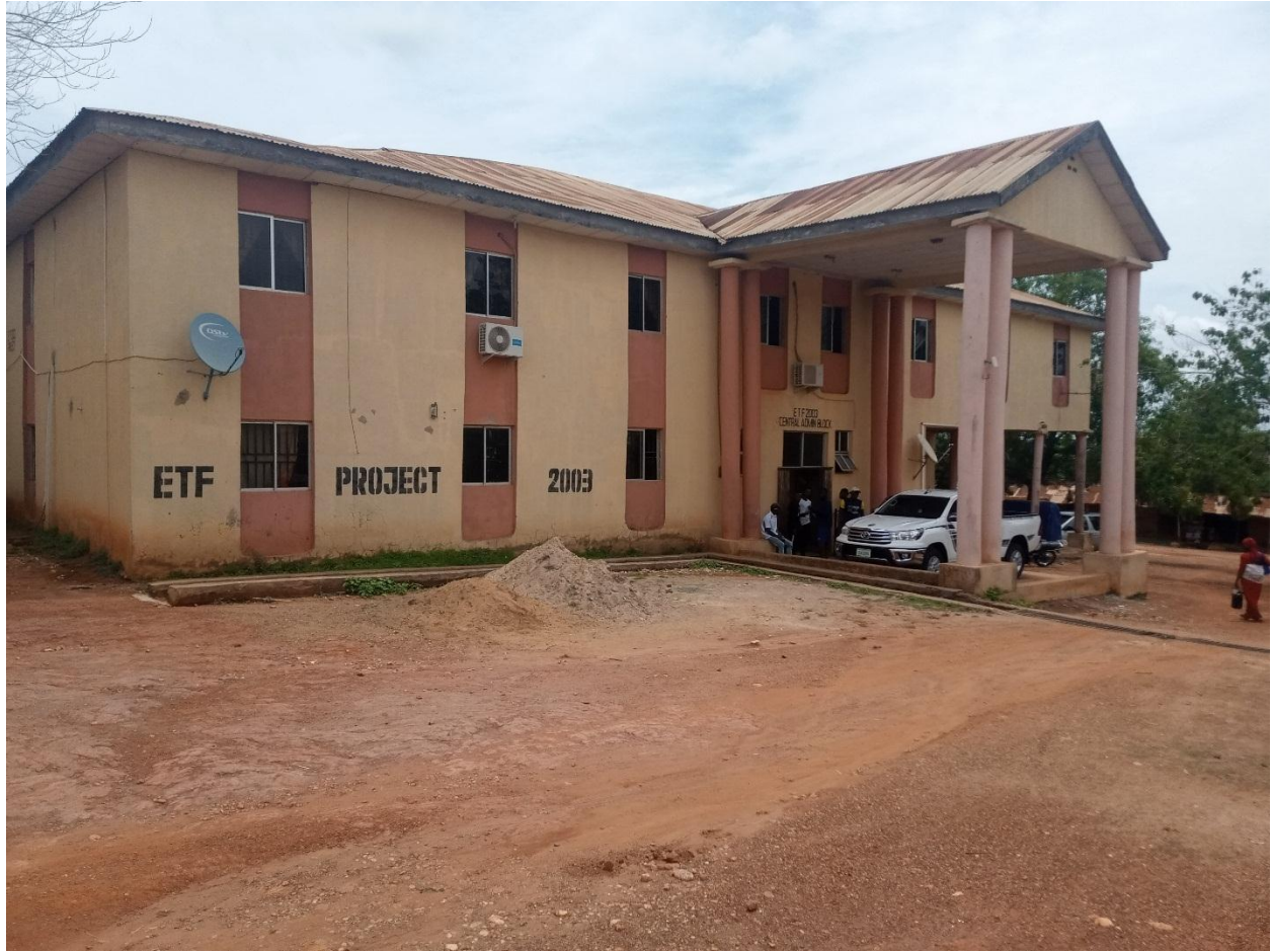
ETF 2003 Administrative Block
